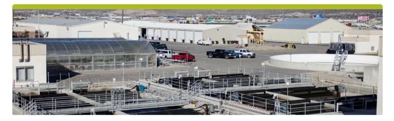
The Spanish Fork City Wastewater Treatment Plant existing facility reached its biological capacity due to changed in the water quality standards, which required nitrification of the waste stream. AQUA Engineering assisted the City as Design Engineer and Construction Management.
