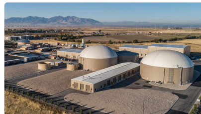
Wasatch Resource Recovery Resource Recovery Facility
