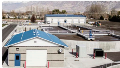
City of Orem Wastewater Treatment Facility
